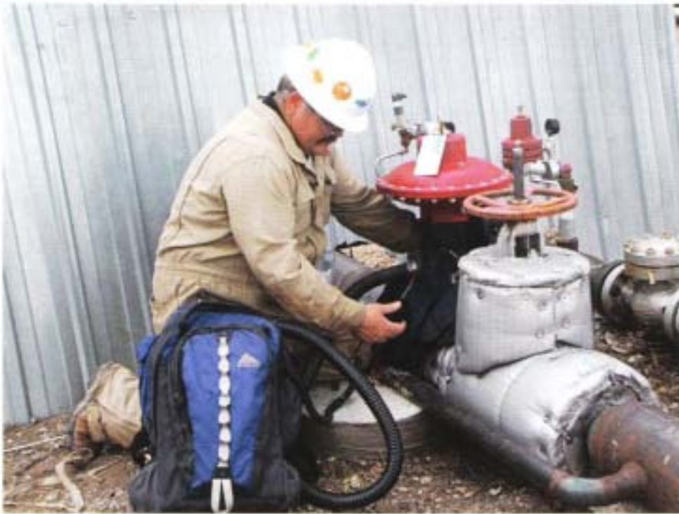
Hy-Bon Engineering's Identify, Quantify, Rectify (IQR) Manager Butch Gidney uses a high flow sampler to quantify a gas leak.
